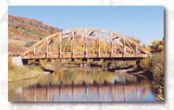
The three-pin arch and the bowstring truss offer a striking combination of wood and steel. The panelized timber deck system shortens construction time. Crash-tested railings and asphalt wear surface provide the performance expected with modern vehicle bridges.
